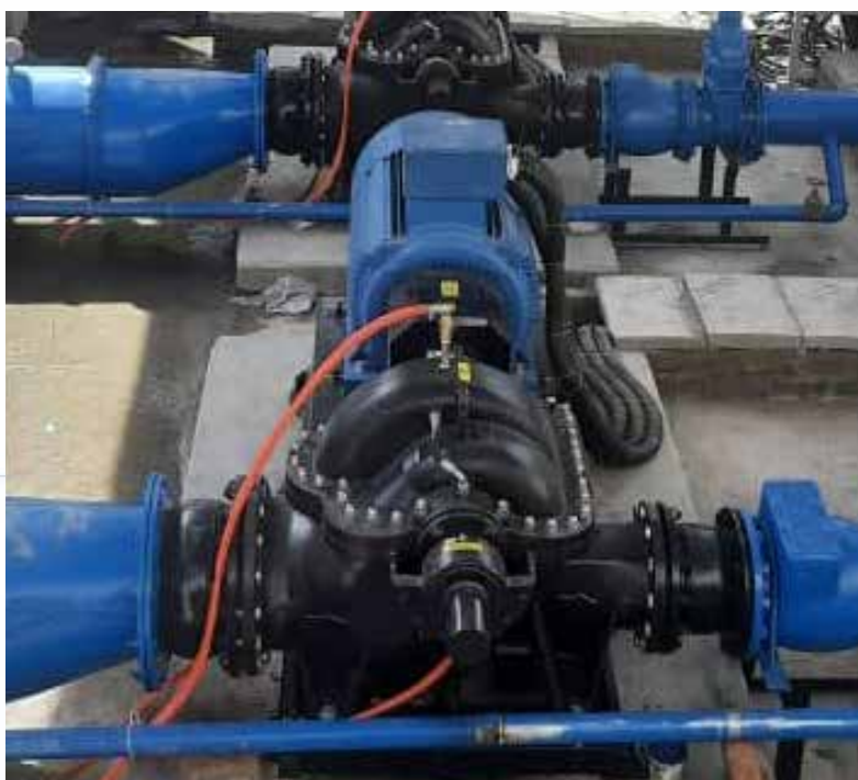
NR. 5 SKDW-4P 250-400 200kW AFGHANISTAN ONE OF THE LARGEST PUMPING STATIONS POWERED BY PHOTOVOLTAIC PANELS IN THE WORLD
